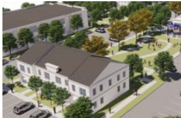
Fig 1.5: Townhomes & 2-story residential buildings in redeveloped Sierra Plaza
