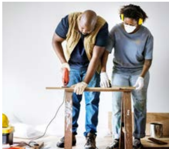
Fig 4.31: Home Renovation Source: www.google.com
